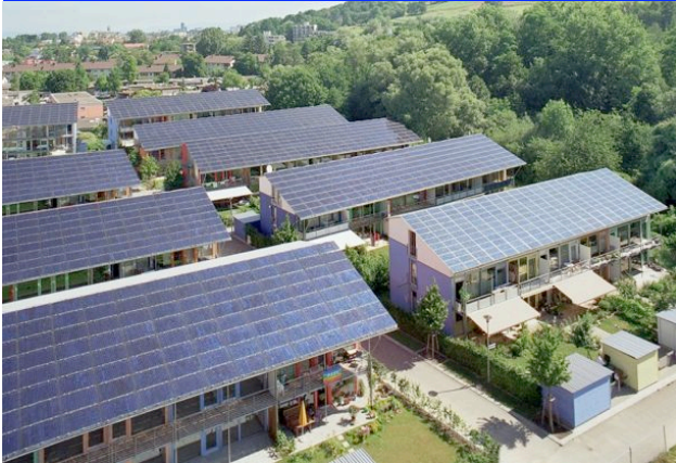
Vauban solar suburb
