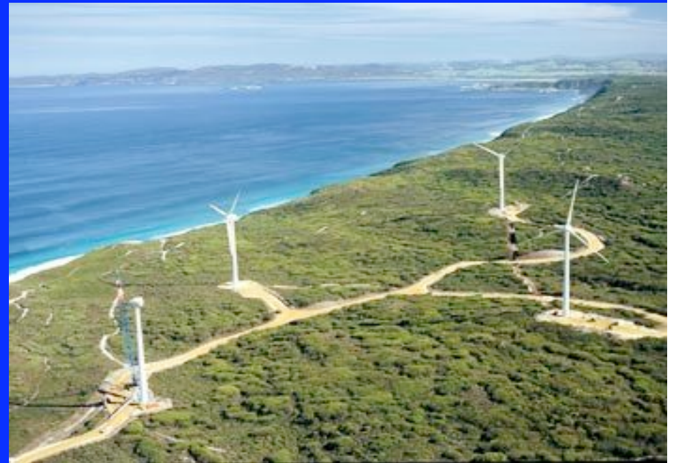
Albany wind farm, Western Australia.
